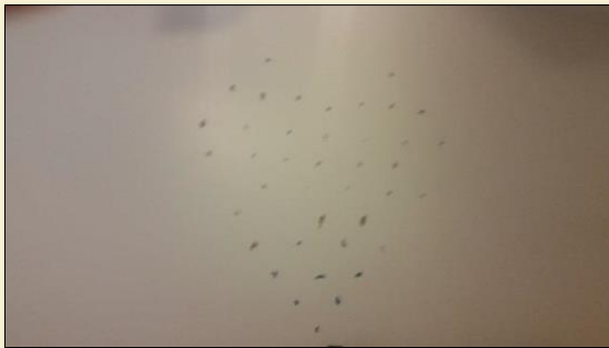
Wall damage examples – minimum $50 charge
