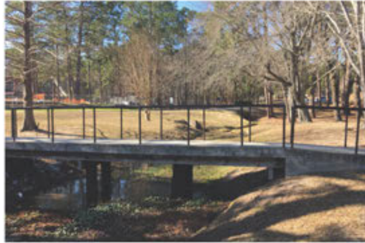
Bridge across Ezra Pond.
