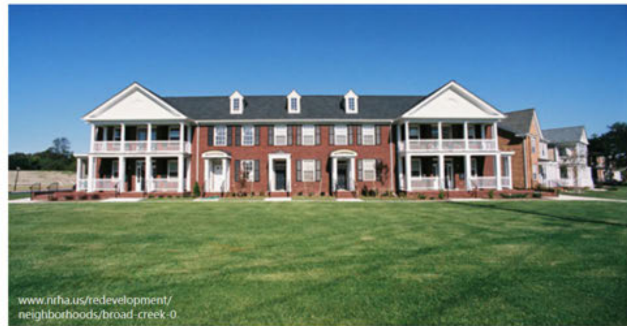
View of townhomes from the front.
