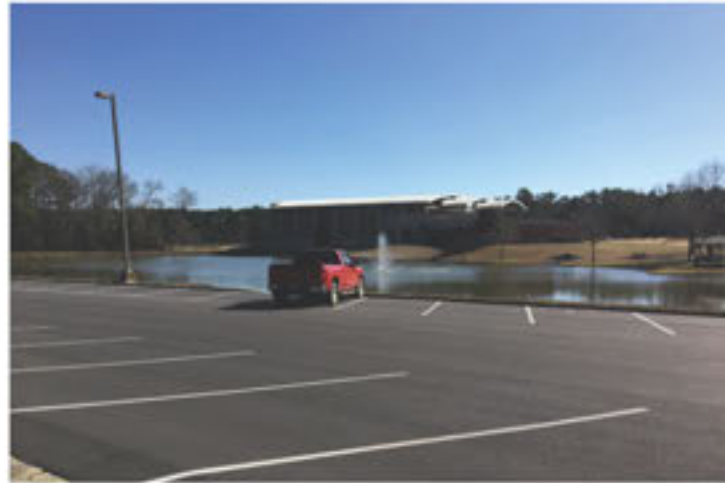
Parking lot below Bobcat Villas allows runoff to go swiftly into Ezra Pond.
