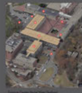
Existing Science Center (Shapiro Center)
